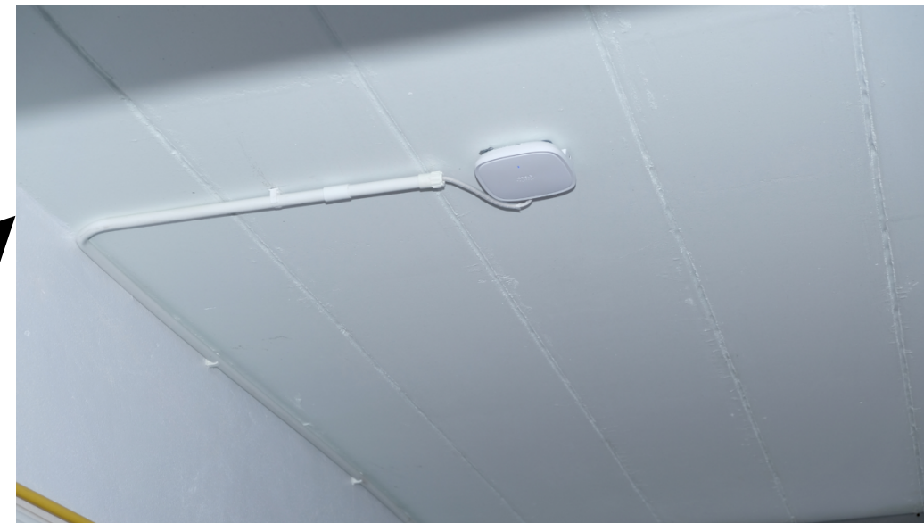
router, via WiFi
